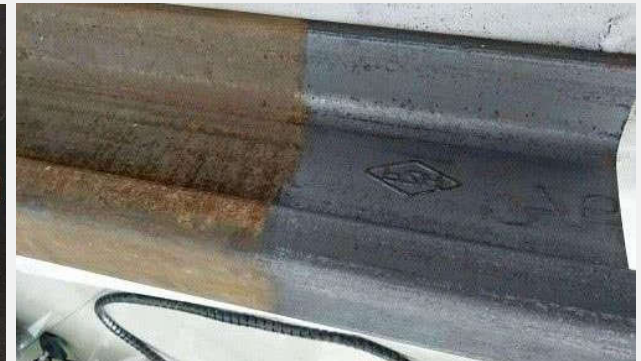
Railway track derusting
