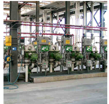
Truck loading bay
